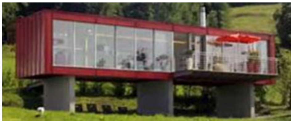
Cargo containers converted to living units.
